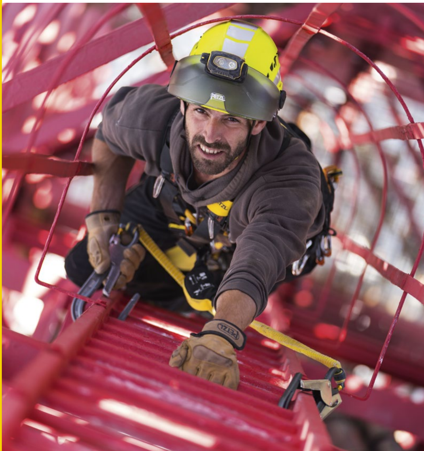
Pylone inspection and maintenance © Petzl - vuedici.org - Profil - TDF
