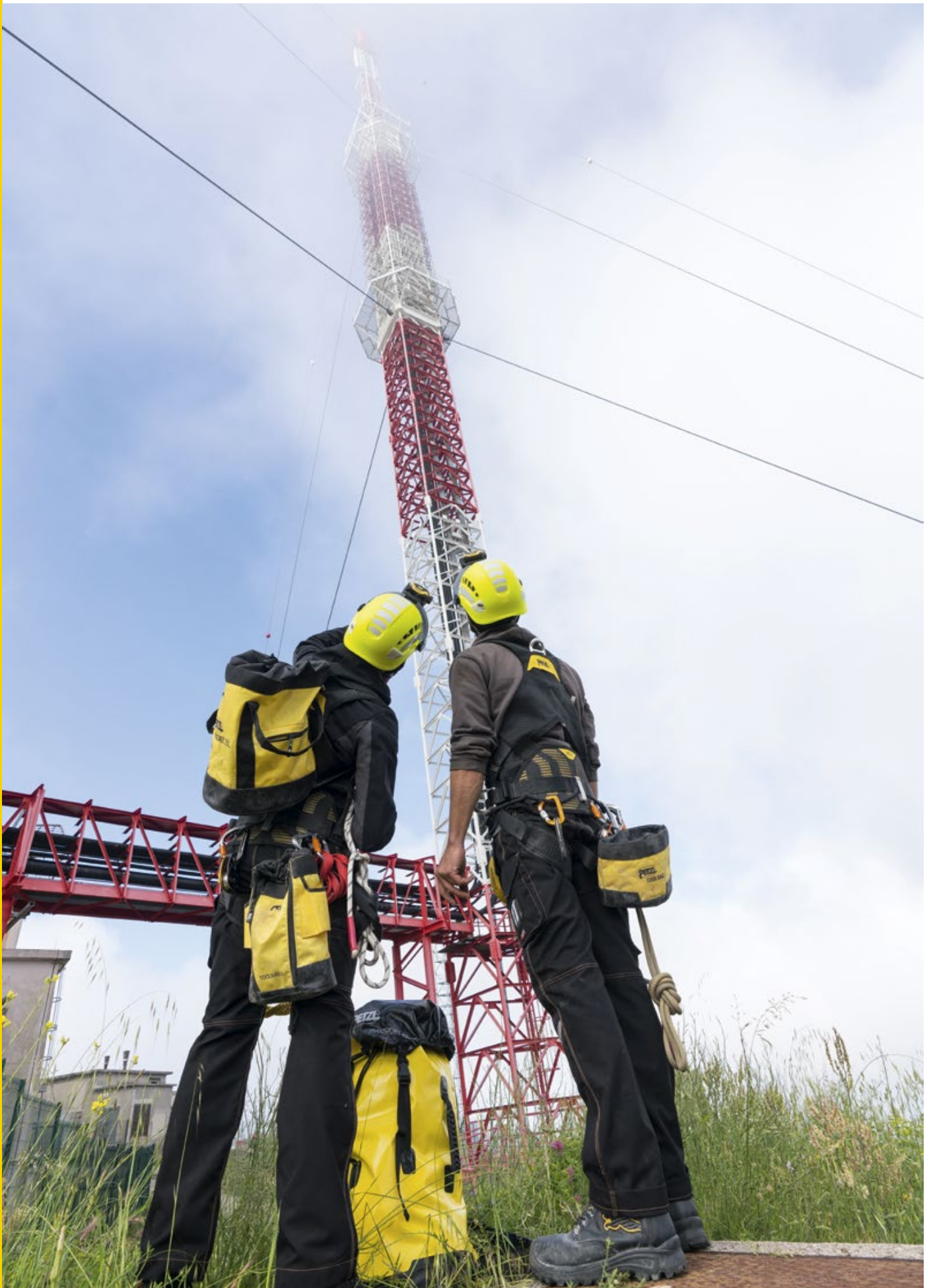
Pylone inspection and maintenance © Petzl - vuedici.org - Profil - TDF
