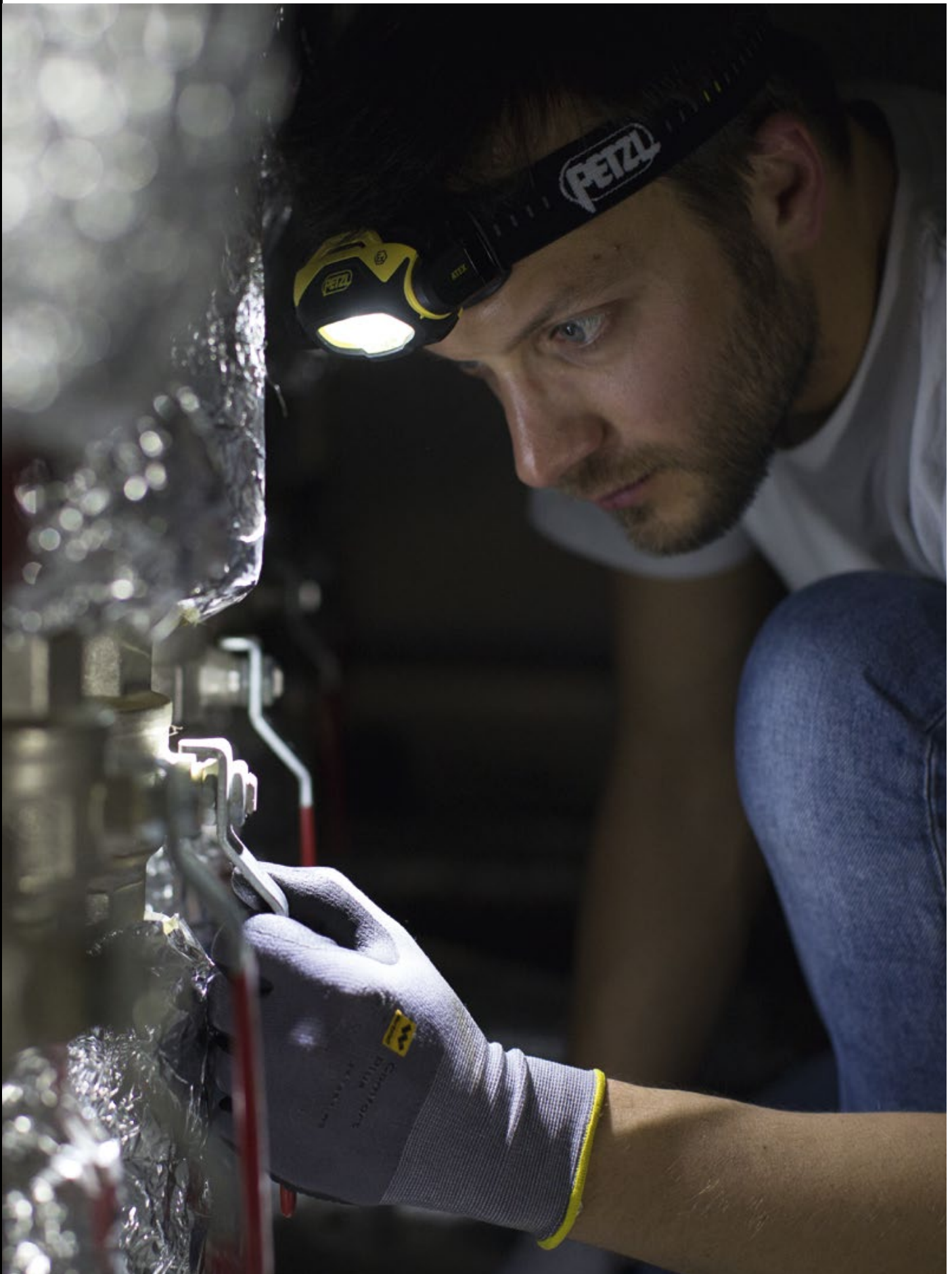
Boiler room inspection and maintenance © Petzl - Lafouche
